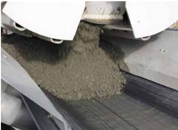
Figure 5.3.1: Production of Roller-Compacted Concrete
