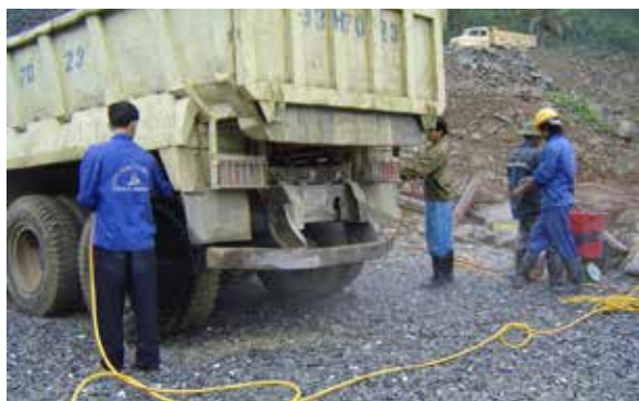
Figure 5.4.2.2: Workers wash a haul truck's tyres to prevent contamination of lift surfaces
