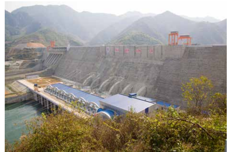
Figure 3.2.1.1: A completed RCC dam
