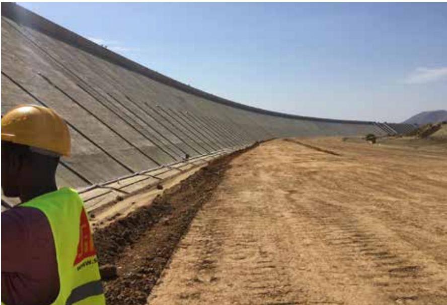
Figure 6.1.1: A saddle dam under construction in Africa
