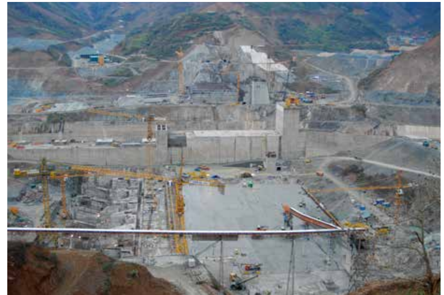
Figure 6.2.1: Surface preparation prior to RCC placement
