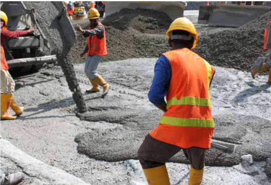
Figure 5.7.2.1: Laying and spreading of bedding mortar
