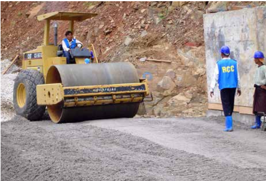
Figure 3.1.1: The RCC under compaction
