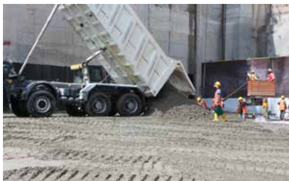
Figure 5.4.2.1: A truck unloads RCC at dam site
