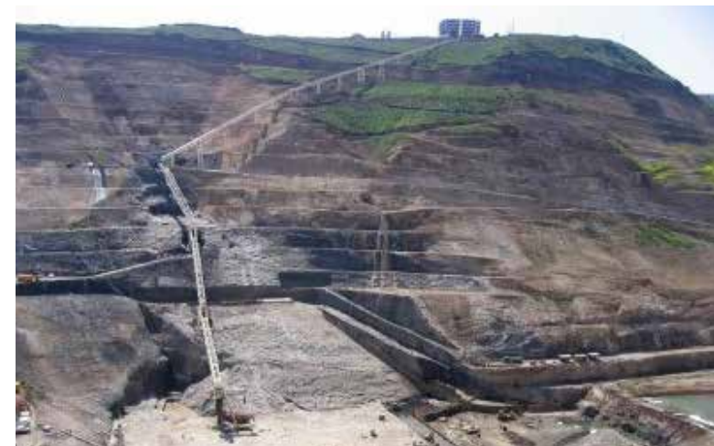
Figure 5.4.1.1: A conveyor system transports RCC from the top of a mountain to the dam site
