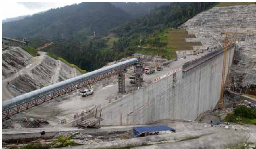
Figure 1.2.1: RCC dam construction
