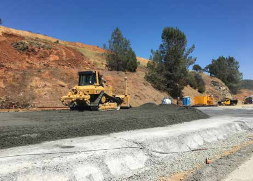
Figure 3.2.2.2: RCC spreading
